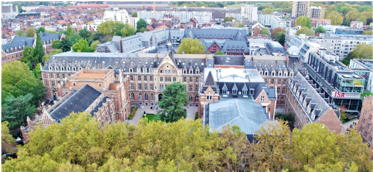
Figure 3-12 Bird's eye view of the JUNIA-ICL demo site.
